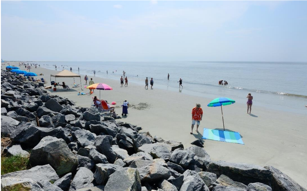
Figure 16.100 The Broad Beach Riprap is Designed to Retain Sand. Image by Ralph Daily, CC BY 2.0.
