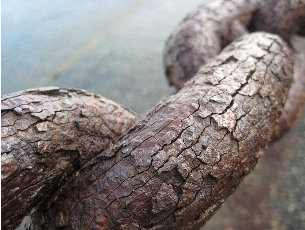
Figure 12.64 Example of Rusting- or Oxidation on the links of a chain near the Golden Gate Bridge in San Francisco ; it was continuously exposed to moisture and salt-laden spray, causing surface breakdown, cracking, and flaking of the metal. Image is used under a Attribution-Share Alike 3.0 Unported license.
